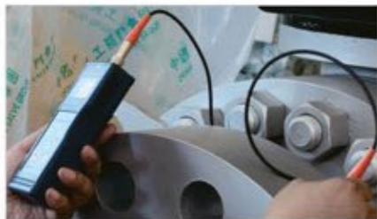
Ultrasonic Thickness Measurement
